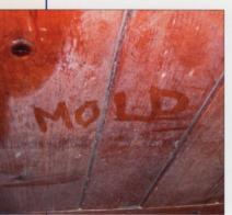
Dirt crawl spaces have the high humidity levels necessary for mold growth. Humidity levels from 50% to 90% are easily found in dirt crawl spaces that have never flooded.
