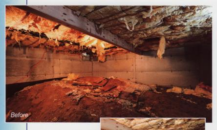
A dirt crawl space under a home is a very bad idea. The earth has very high humidity in the soil. This water vapor moves easily into the crawl space and upwards into the house environment.
